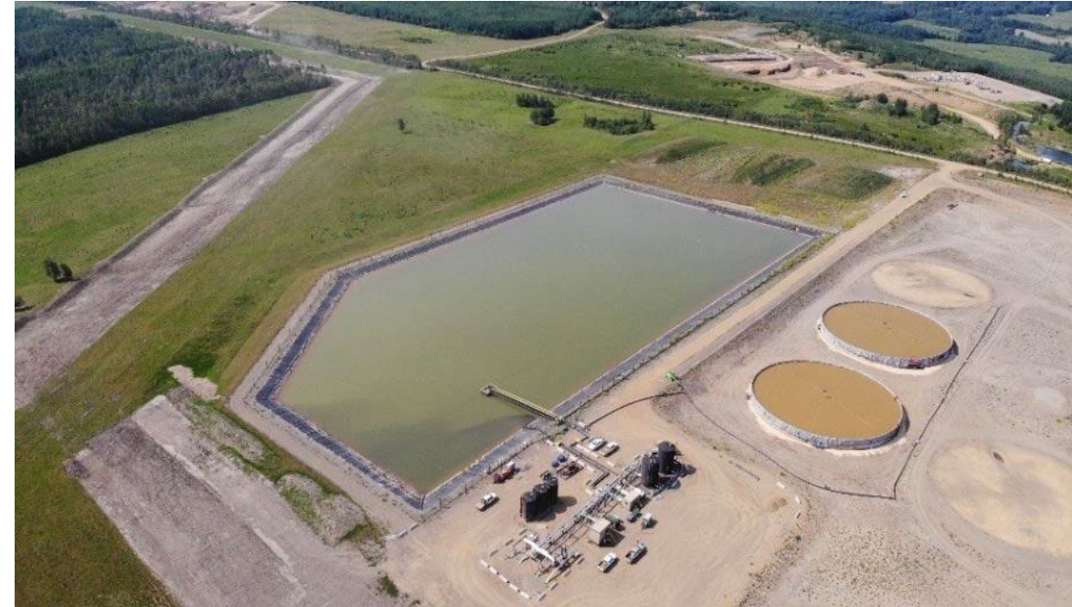
Tupper Montney Produced Water Pond
