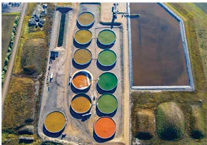
Produced water pond and facility in the Tupper Montney.
