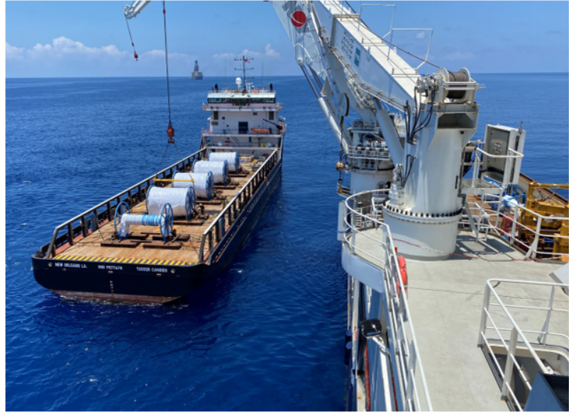
King's Quay Mooring Line Installation
