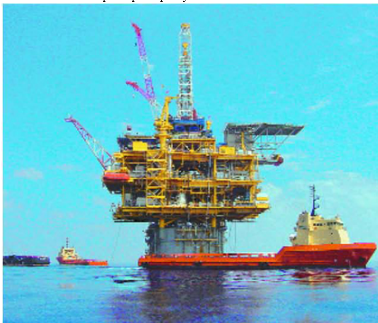
The first well at the Front Runner field in Green Canyon Block 338 began producing through this spar facility in December 2004.
