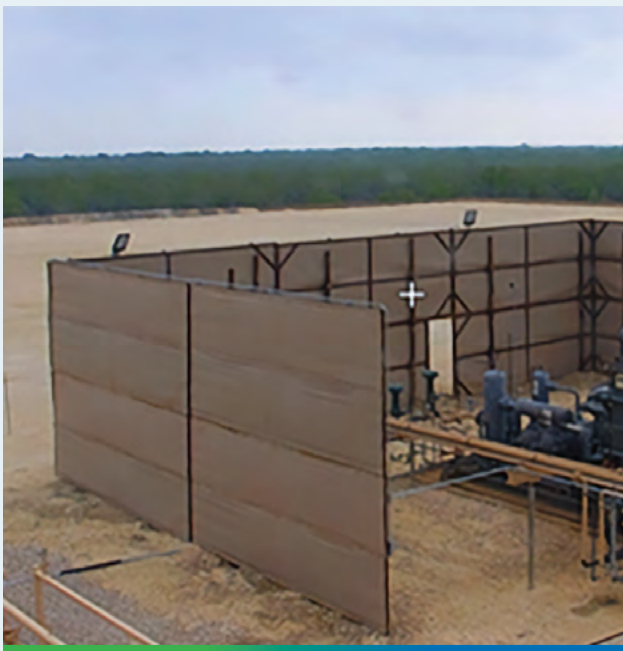
Sound barrier installation at Eagle Ford Shale
