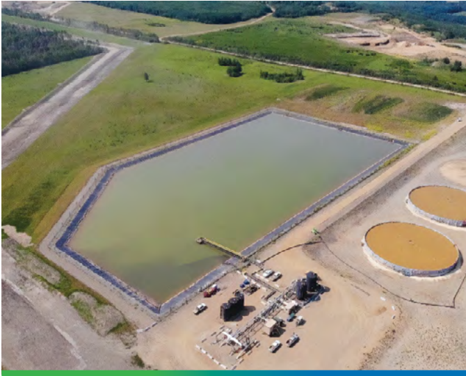
Produced water pond and facility in Tupper Montney.
