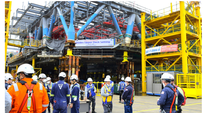
Fabrication of King's Quay in the Hyundai Heavy Industries Yard in South Korea
