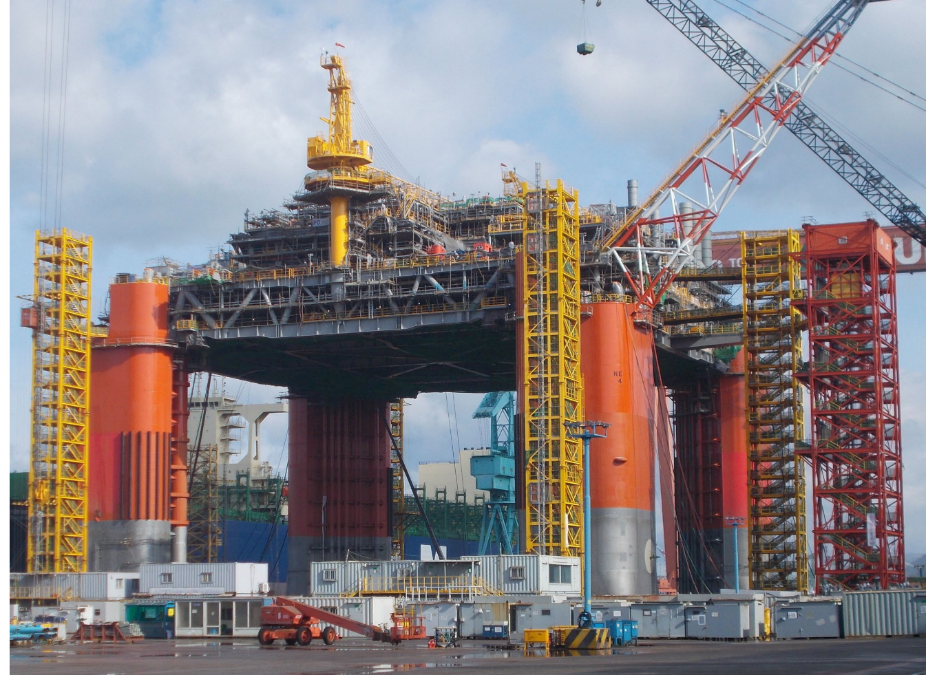
King's Quay – Platform Crane Installation
